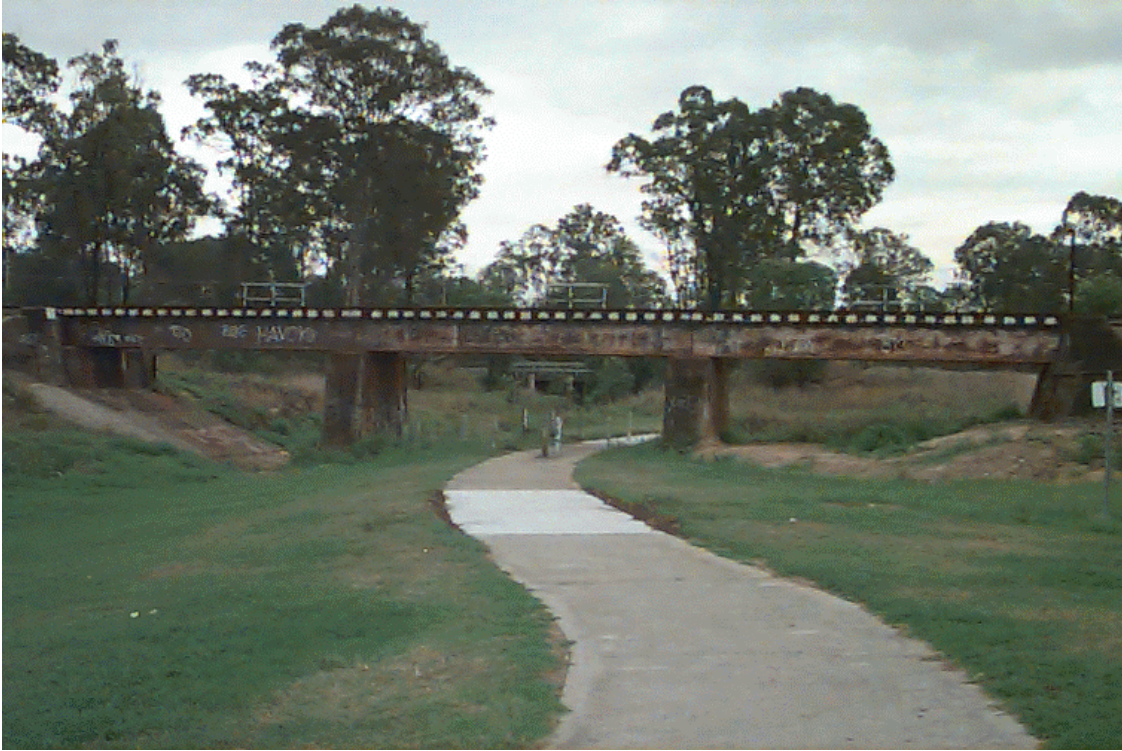
Railway Crossing, 1997 facing downstream
