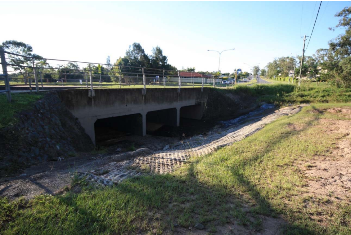
Algester Rd North Crossing, 2015 facing downstream
