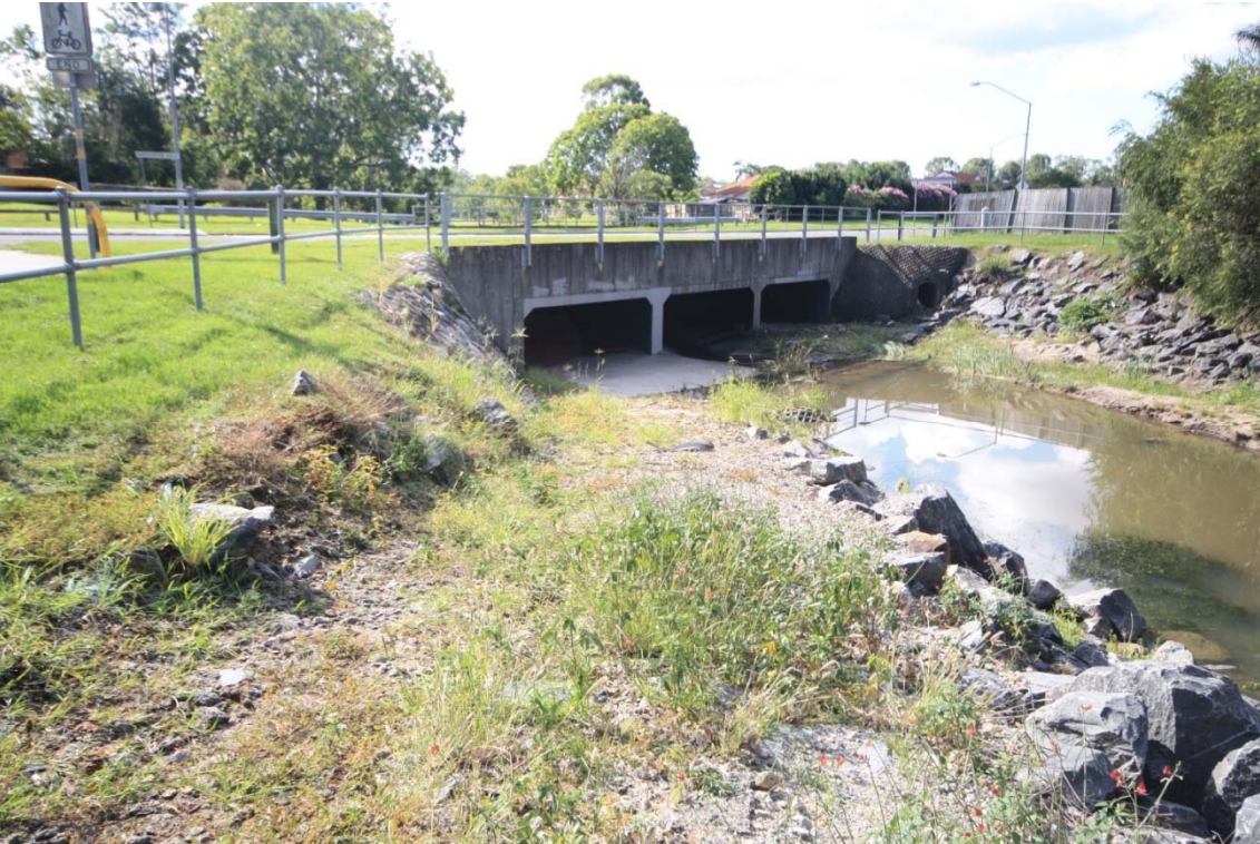
Algester Rd South Crossing, 2015 facing downstream
