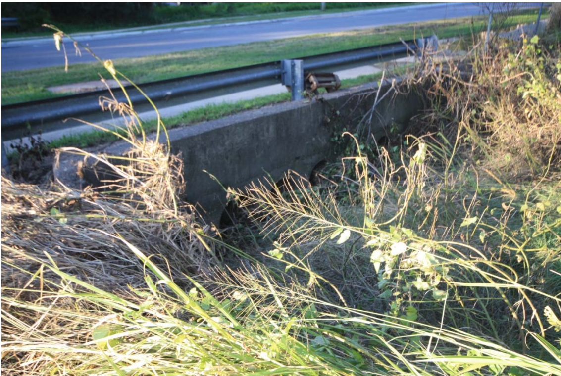
Formby St Crossing, 2015 facing downstream
