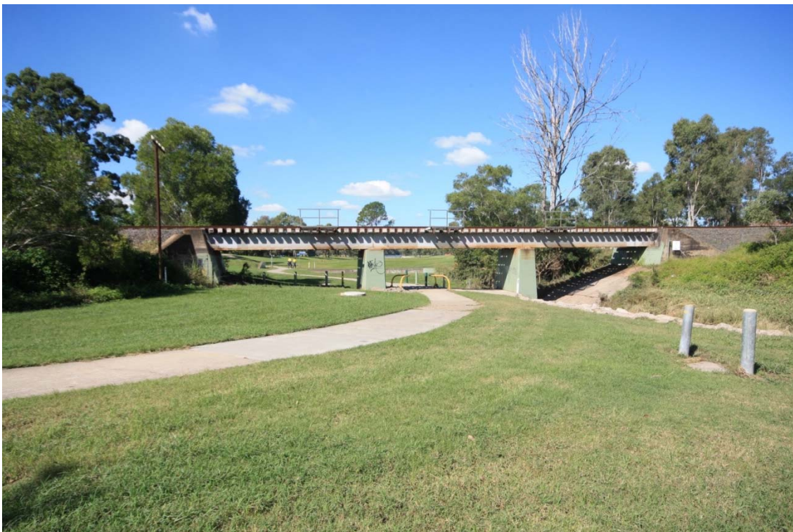
Railway Crossing, 2015 facing upstream,
