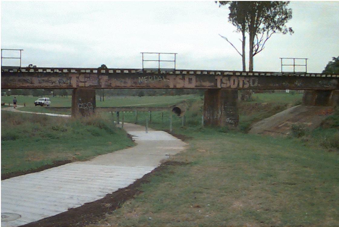
Railway Crossing, 1997 facing upstream
