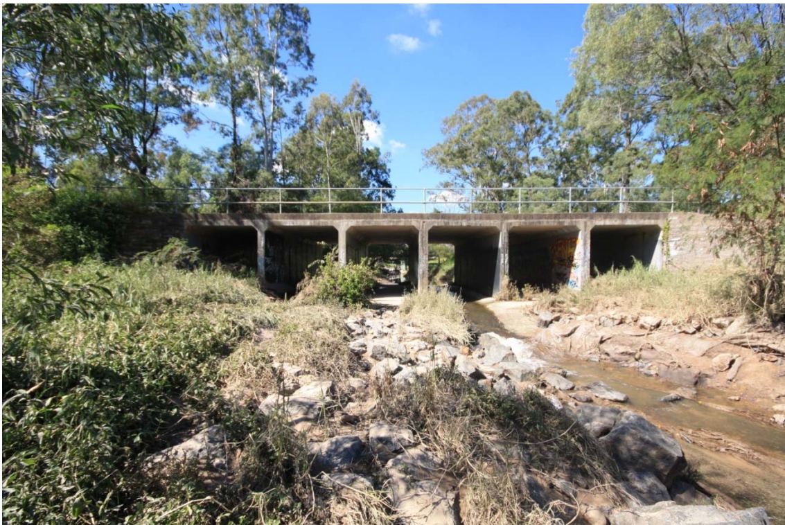
Paradise Rd Crossing, 2015 facing upstream
