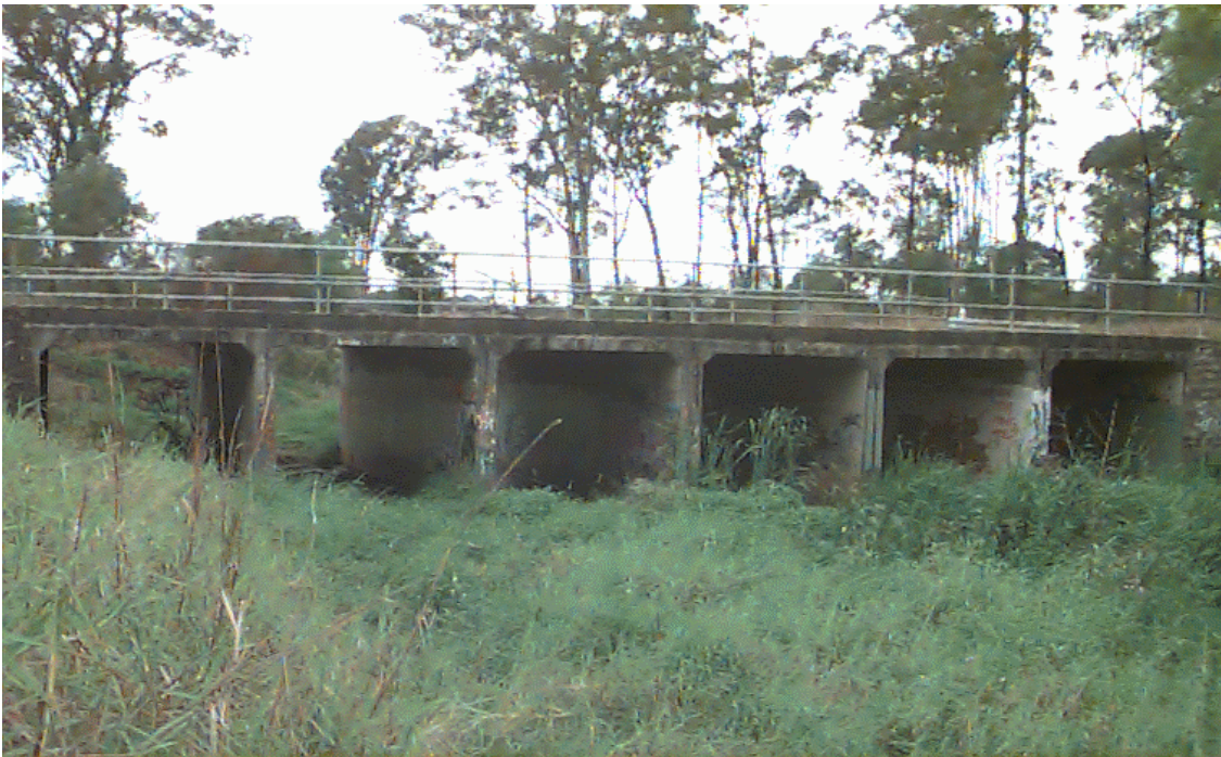
Paradise Rd Crossing, 1997 facing upstream
