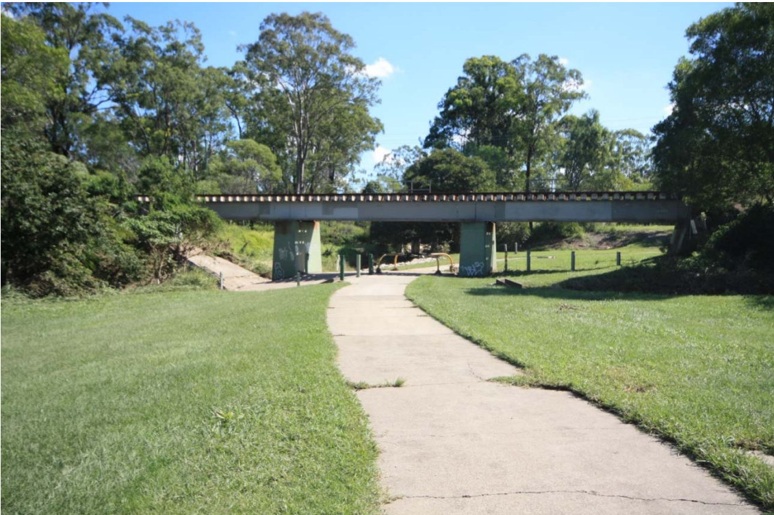
Railway Crossing, 2015 facing downstream
