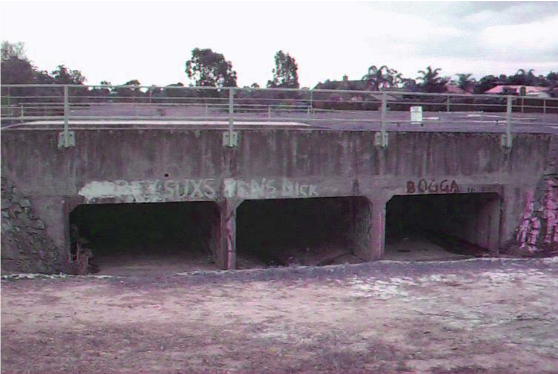
Algester Rd North Crossing, 1997 facing downstream
