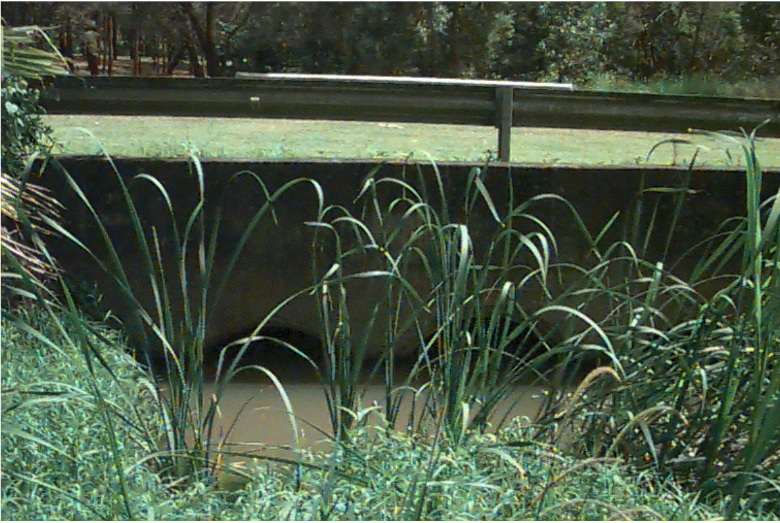
Ormskirk St Crossing, 1997 facing upstream
