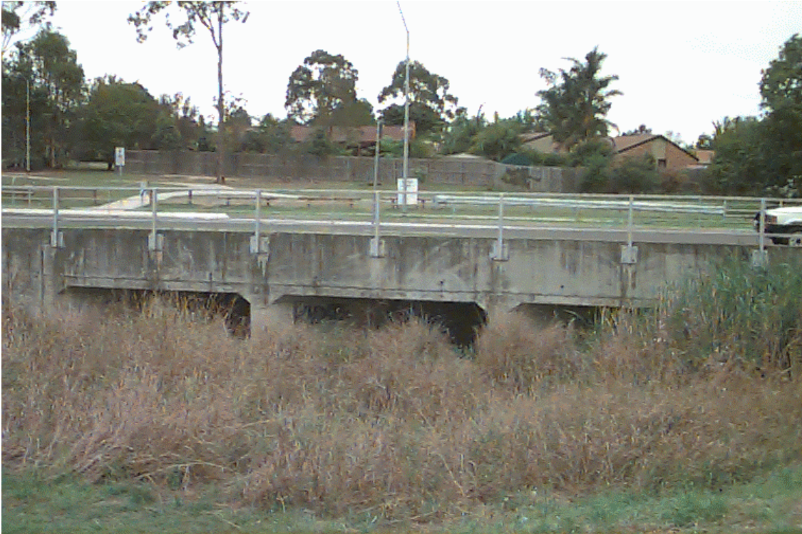
Algester Rd South Crossing, 1997 facing downstream
